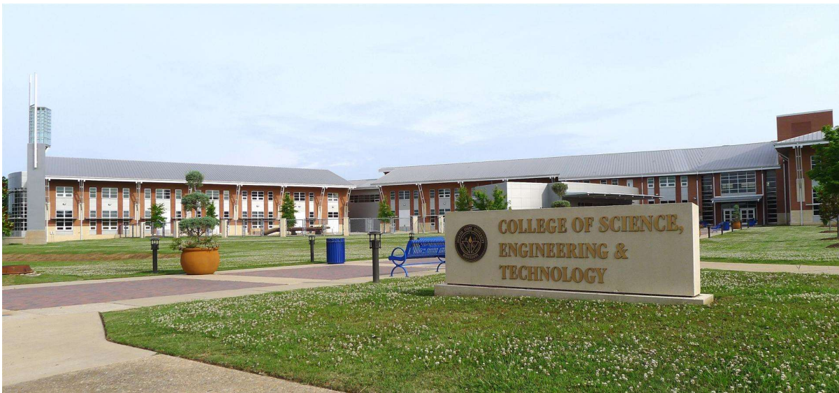
Figure 7-1. Front view of the new Engineering Building
